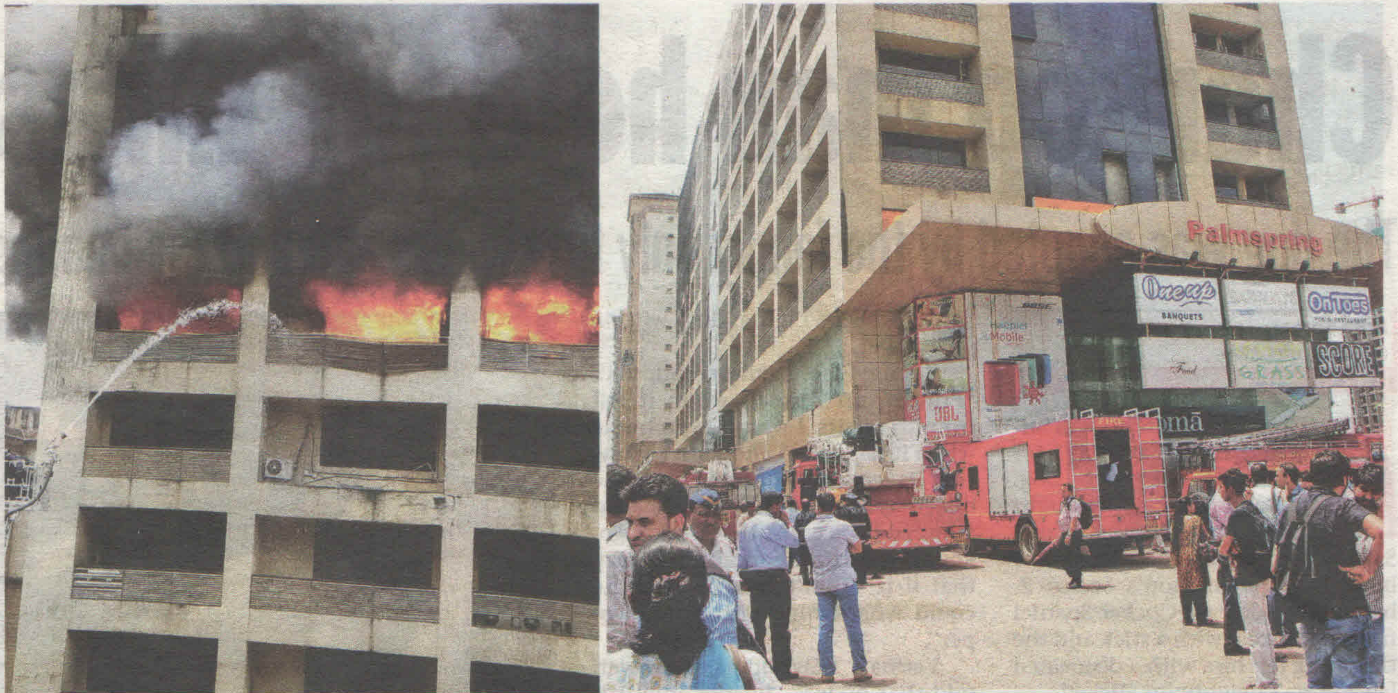
The Palm Springs building on the Link Road in Malad (W) had serious safety lapses, the firefighters said
